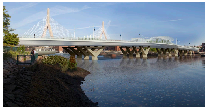
Figure 11. Proposed Bridge Elevation Showing V-Piers Reflecting the Pyloos of the Zakim Bridge (Rendering)
