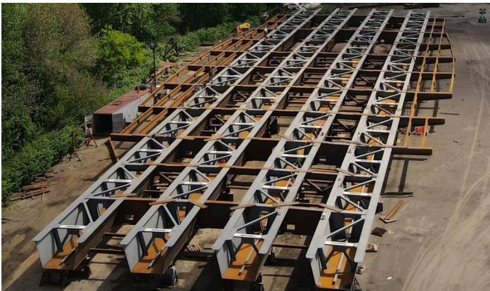
Figure 4 Fit-up of Span 7 Steel Framing in Construction Yard
