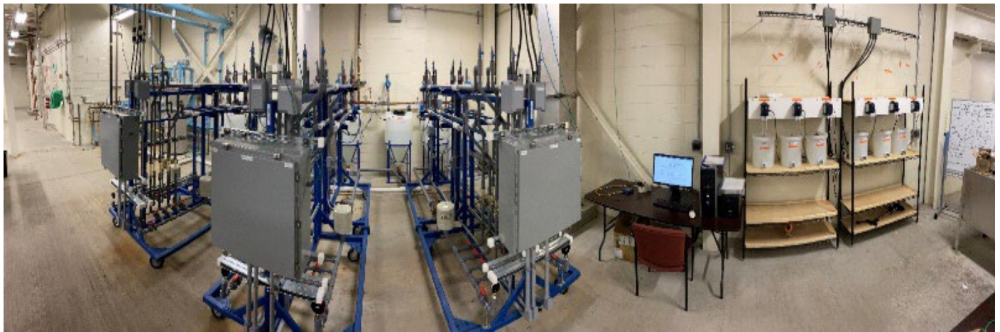
Figure 8. Corrosion control study - lead pipe rigs.
