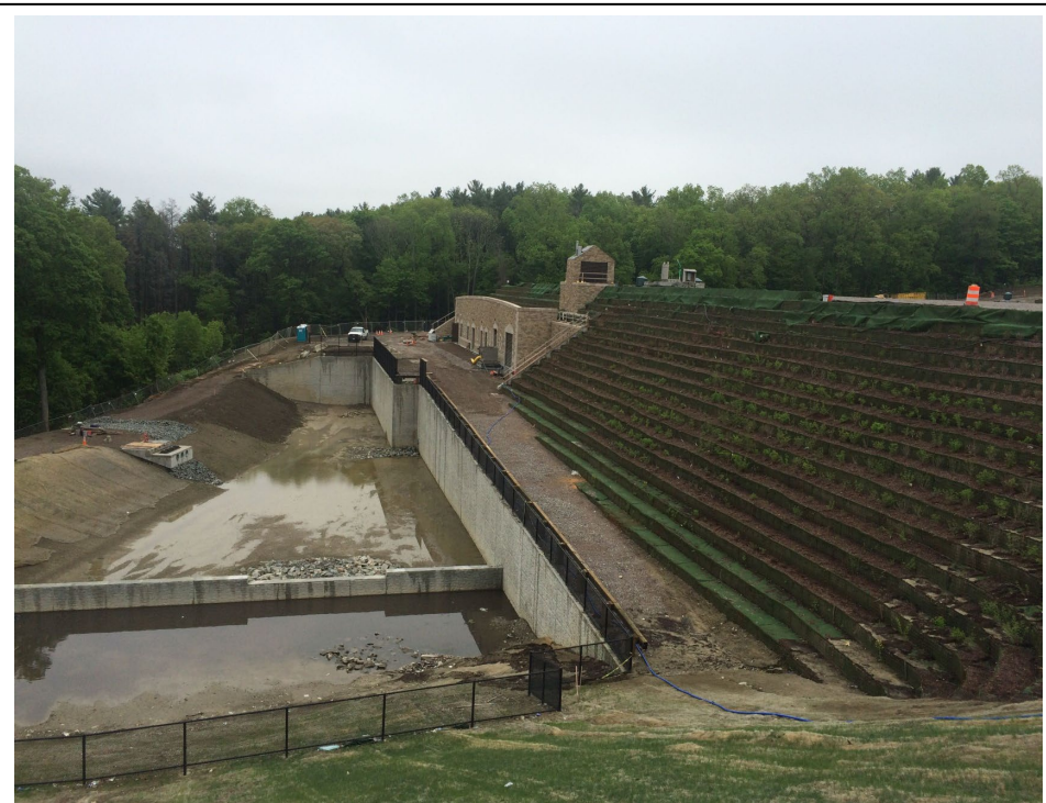
Figure 6. Spot Pond Pump Station and Storage Tank project (MWRA 2004-2015)
