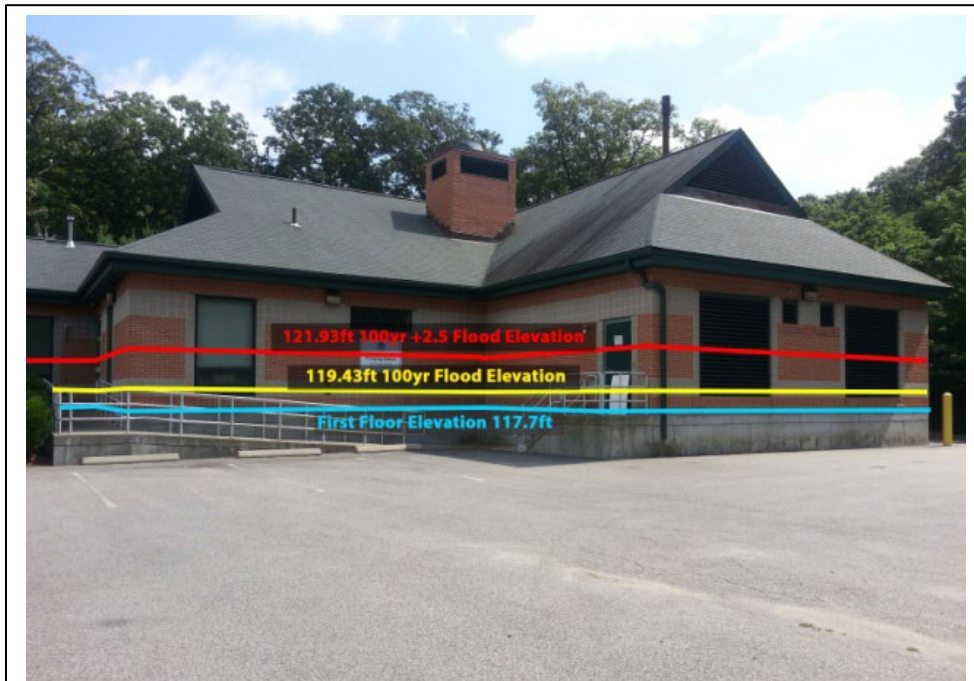
Figure 2. Quincy Pump Station flood line scenarios drawn to represent water levels at two different benchmarks, FEMA 100-year and 100-year +2.5 ft (MWRA, 2016)
