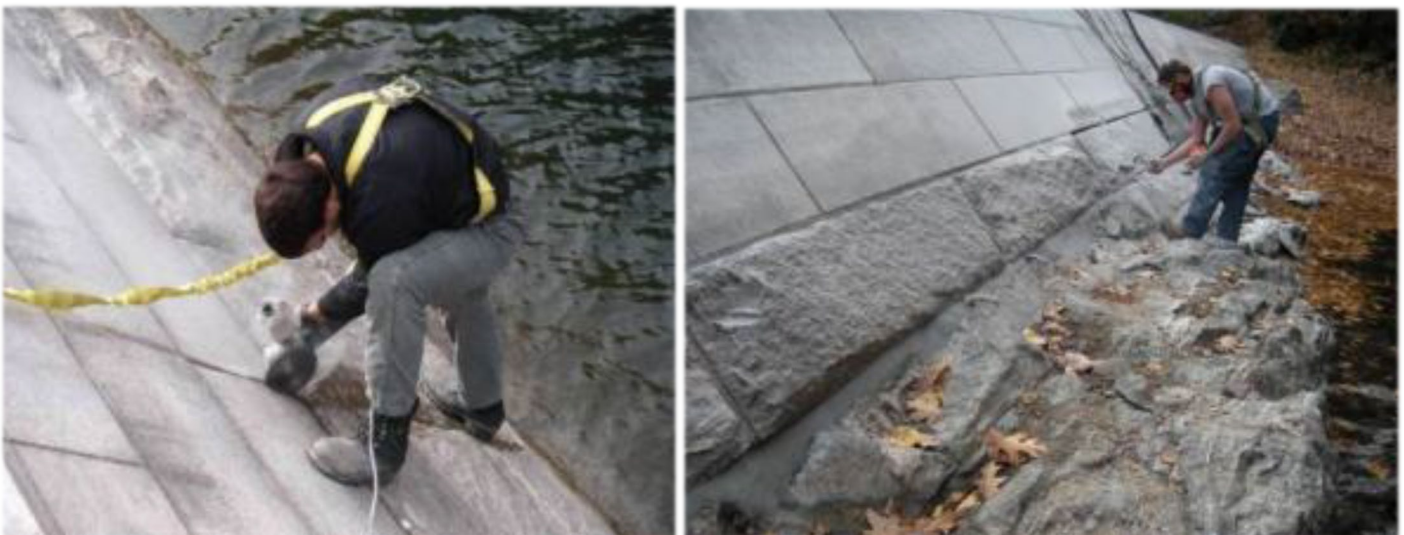
Figure 11. Quabbin Spillway masonry repairs in 2010
