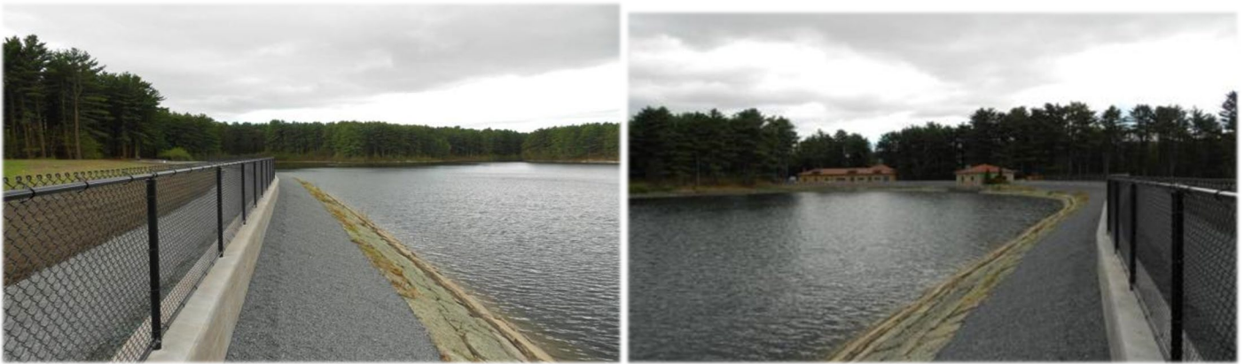
Figure 9. Weston Dam Parapet Wall
