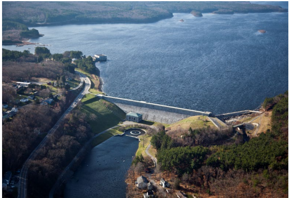
Figure 6. Wachusett Reservoir Dam and Spillway
