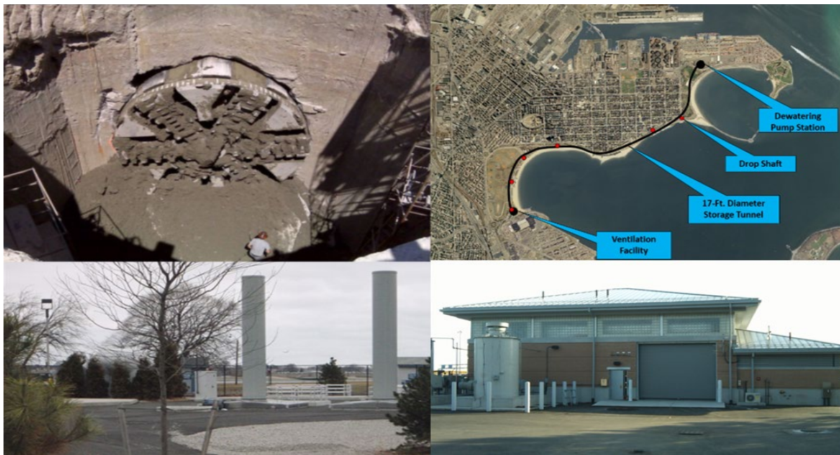
Figure 4. North Dorchester Bay / South Boston CSO tunnel construction and facilities (MWRA 2004-2015)
