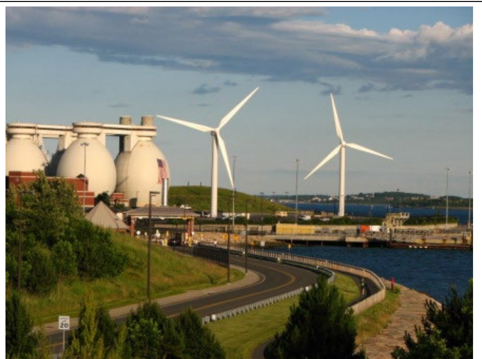
Figure 5. Deer Island view from public access looking south. Egg-shaped digesters (the heart of Deer Island's green energy program), and its two wind turbines (MWRA, 2023).
