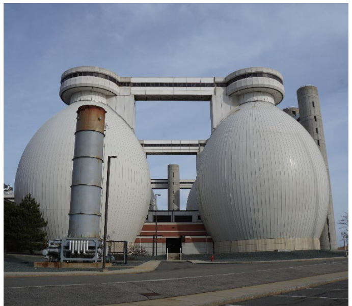
Figure 4. Two of the twelve digesters at Deer Island (MWRA 2023).
