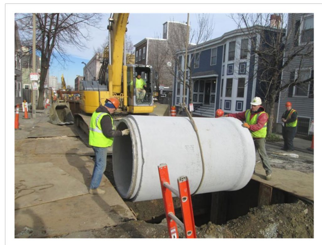
Figure 3. Stormwater drain construction to support sewer separation (MWRA 2004-2015)
