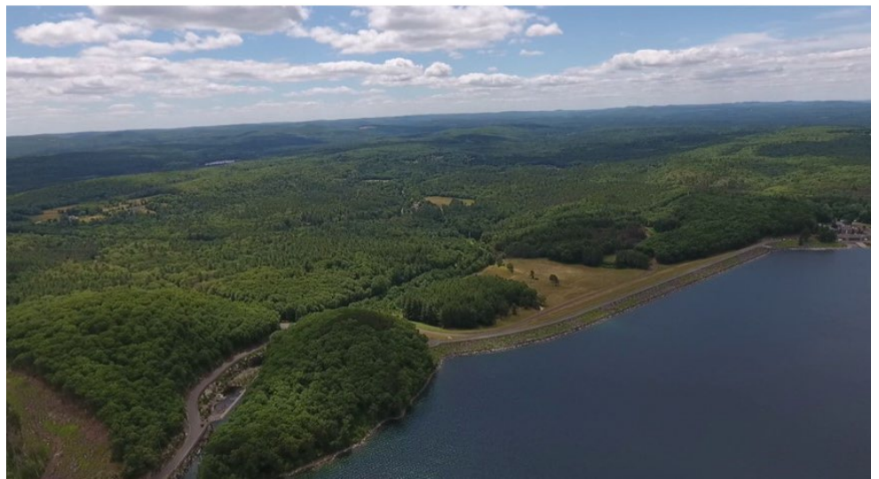
Figure 5. The massive Winsor Dam looking downstream from Quabbin Reservoir
