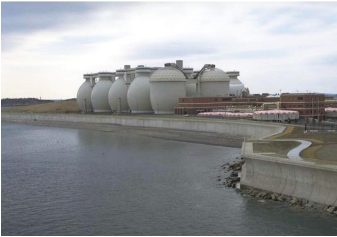
Figure 1. Deer Island Treatment Plant is protected for 100-year flood, 1.9-foot sea level rise, and a wave run-up of 14 feet on its east side and 2 feet on its west side (MWRA, 2023).
