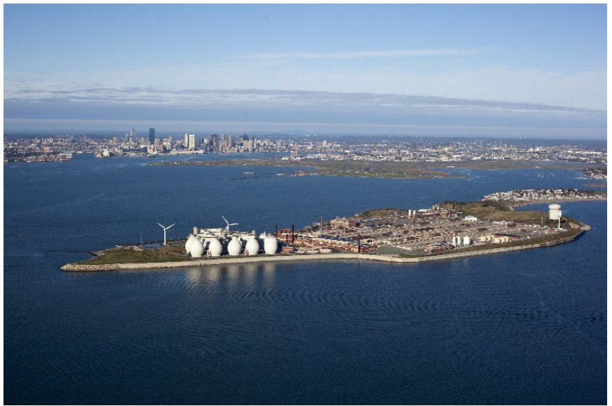
Figure 1: The Deer Island Wastewater Treatment Plant, Boston MA (MWRA, 2023)
