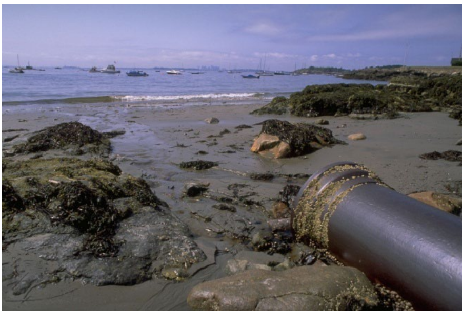
Figure 1. Typical sewer overflow discharging to beach in 1980s (MWRA, 2004-2015)
