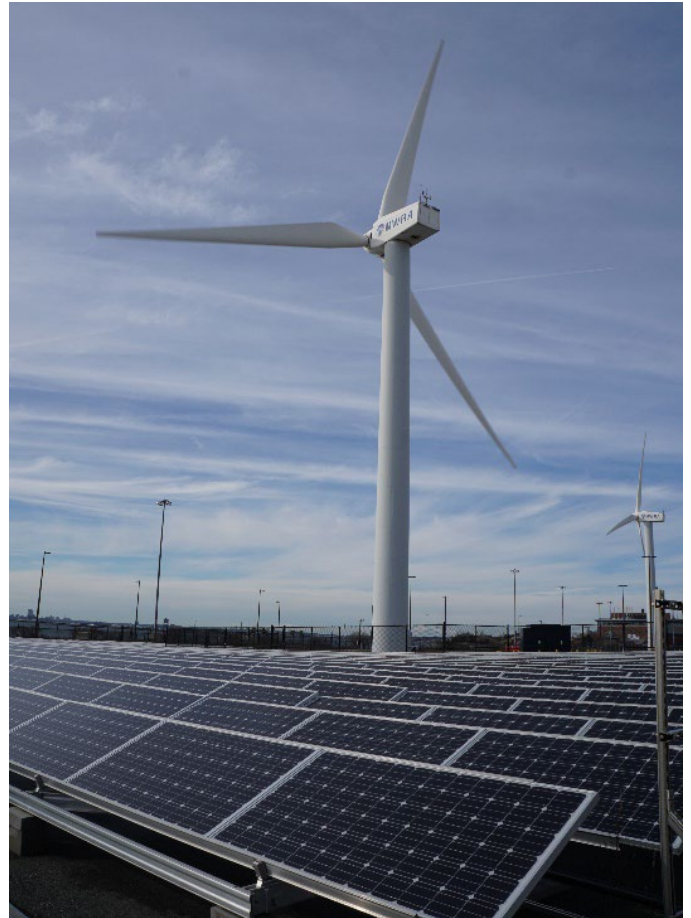
Figure 3. Wind turbine generators and ground mounted photovoltaic array installed at Deer Island (MWRA 2023).
