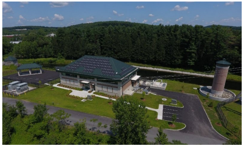
Figure 5. Wachusett Aqueduct Pump Station (MWRA 2004-2015)
