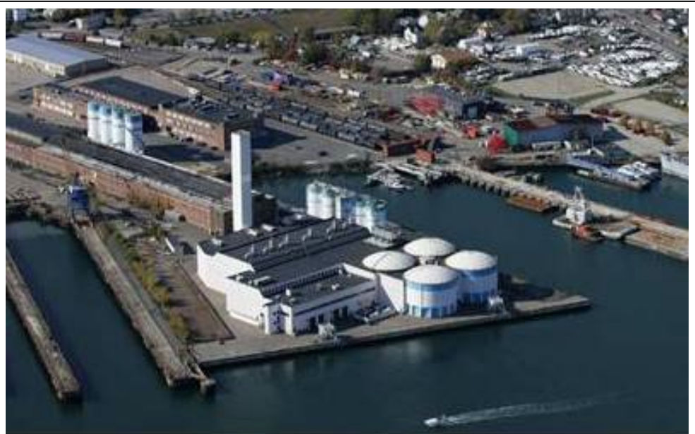
Figure 4. MWRA Pellet Plant, Quincy, MA (MWRA, 2023).
