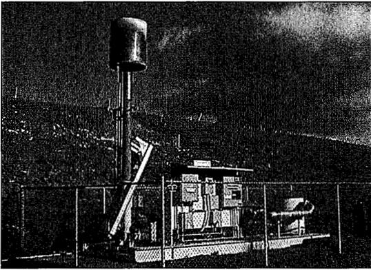
**FIGURE 6.** A typical "candlestick" gas flare installation for the combustion of landfill gas.
