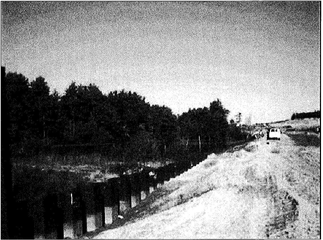
FIGURE 1. A view of a length of the sheet piling.
