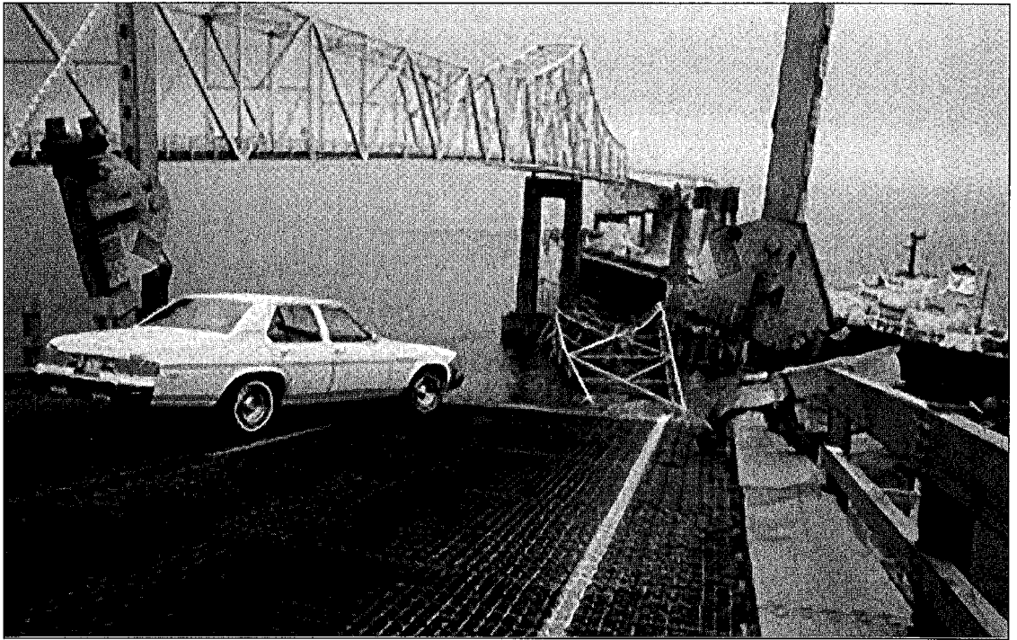
FIGURE 3. The Skyway Bridge after its tussle with a barge.
