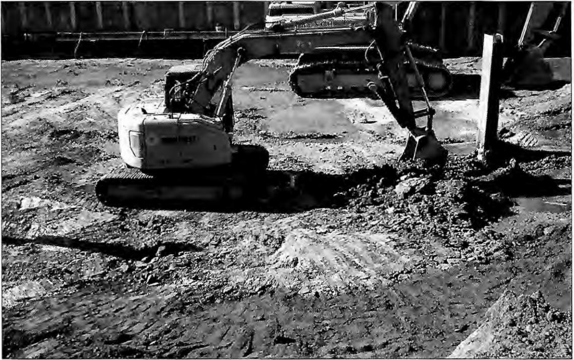
FIGURE 3-96. Gray marine clay under the shovel, covered by reddish-brown organic silty sand in the foreground. (Photo courtesy of Bradford Miller.)
