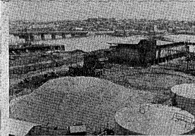
Stage 1 preloading for North tank Excavation for South tank pad
