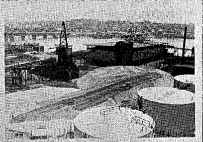
Stage 3 preloading for South tank and transfer to North tank site
