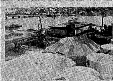
Stage 2 preloading for South tank Gravel pad for North tank placed
