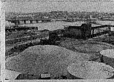
Stage 1 preloading for North tank Excavation for South tank pad
