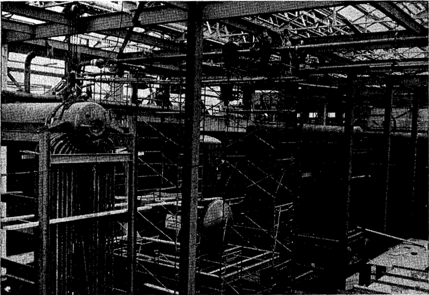
SOUTH BAY INCINERATOR BOILER ROOM—SHOWING ERECTION OF 3 DRUM TUBULAR WASTE HEAT BOILERS—CAPACITY 75,000 LB. PER HR. EACH.
