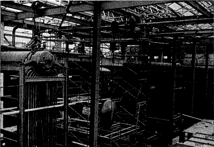
SOUTH BAY INCINERATOR BOILER ROOM—SHOWING ERECTION OF 3 DRUM TUBULAR WASTE HEAT BOILERS—CAPACITY 75,000 LB. PER HR. EACH.
