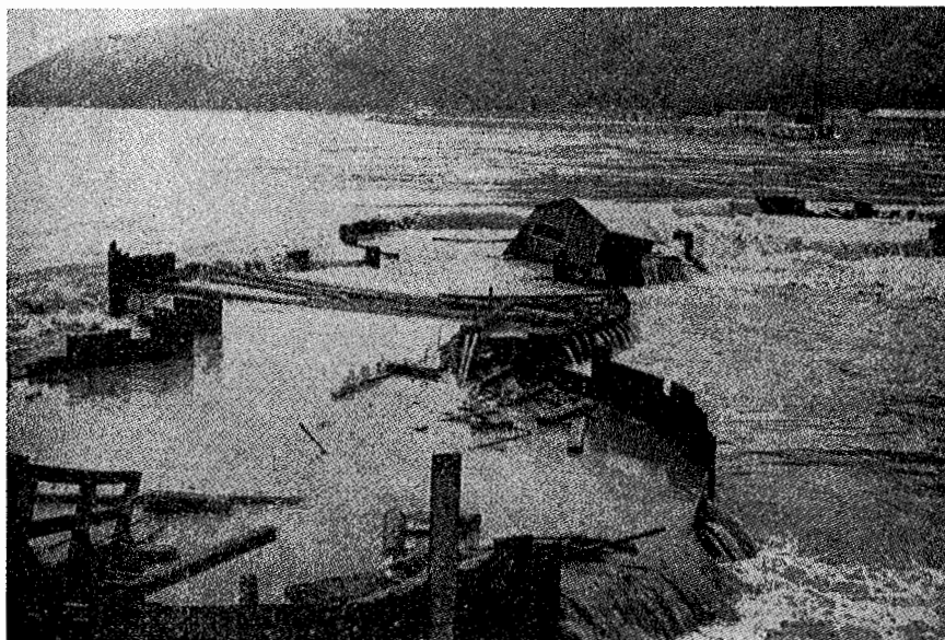
FIG. 7.—FLOODED CELLS OF CONSTRUCTION PIT II DURING JULY 1954 FLOOD.
