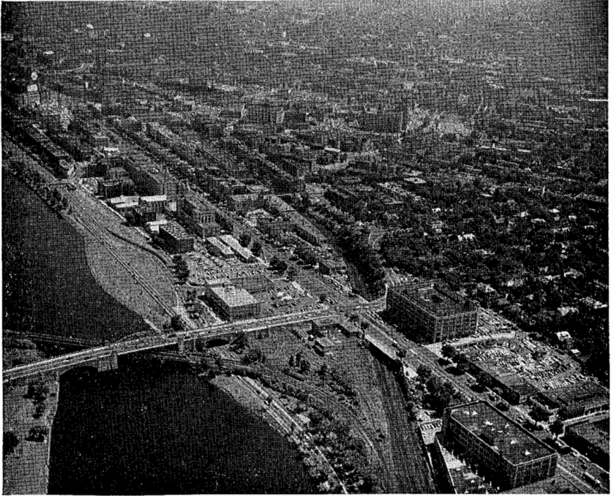
FIG. 3.—AERIAL PHOTOGRAPH OF B.U. BRIDGE AREA.
