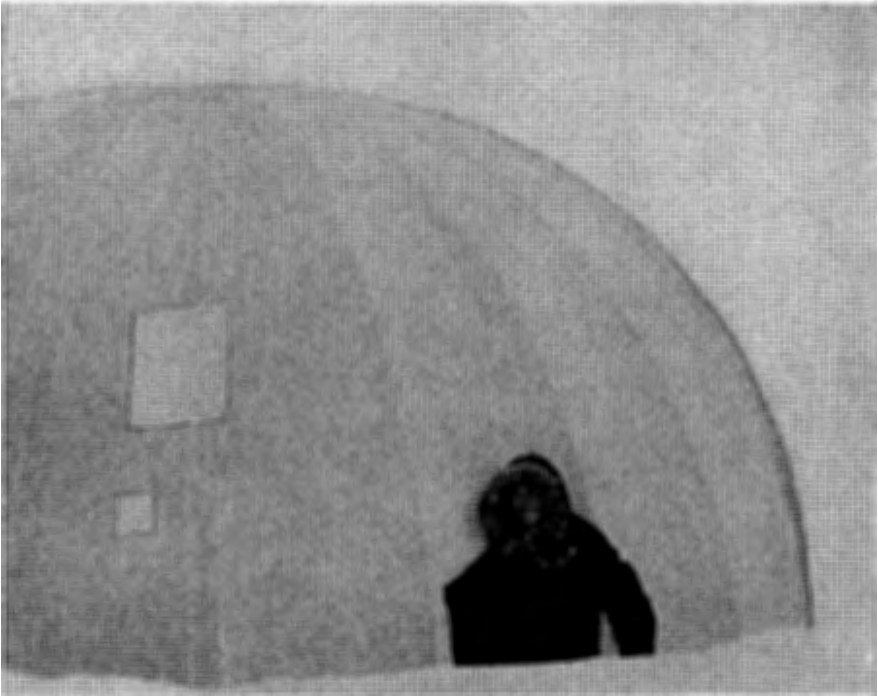
FIGURE 7.—1960 VIEW OF 1953 RADAR SITE.
