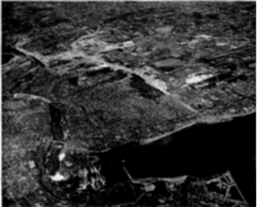
FIGURE 1.—CHIPPEWA-GRASS ISLAND POOL IN RIGHT FOREGROUND WITH CONTROL STRUCTURE AT ITS LOWER END. FALLS AT LEFT FOREGROUND WITH ONTARIO POWER PLANT JUST BELOW CANADIAN FALLS. POWER AUTHORITY CONDUITS PASS DIAGONALLY ACROSS CENTER. (Photo Oct. 21, 1959, courtesy Power Authority of the State of New York.)
