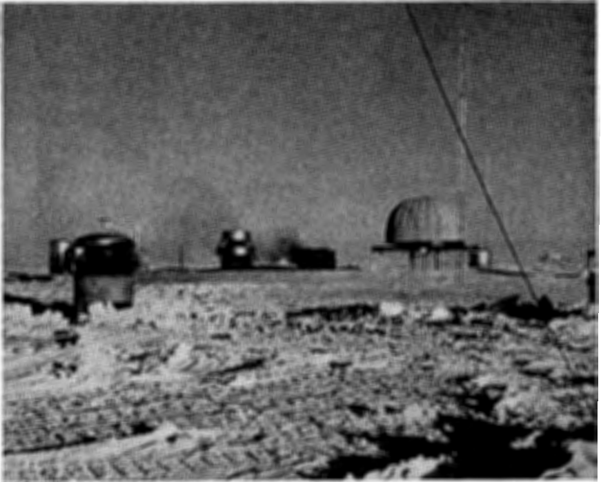
FIGURE 6.—1956 VIEW OF 1953 RADAR SITE.
