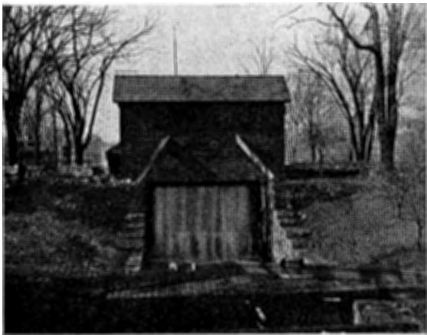
FIGURE 1.—PAWTUCKET CANAL HEADGATES AT LOWELL, MASS., 1956, SHOWING THE "FRANCES GATE" CLOSED AND ADDITIONAL FLASHBOARD PROTECTION.
