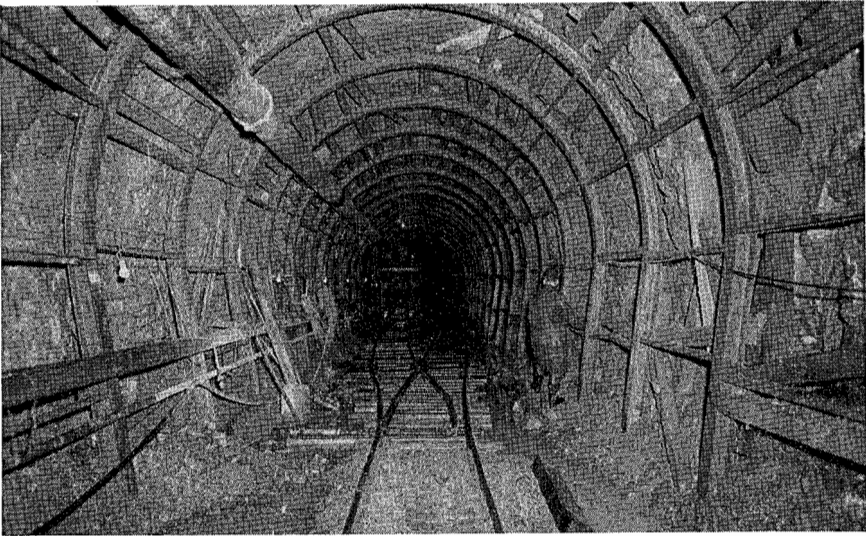
FIG. 11.—LOOKING SOUTHERLY FROM STATION 7 + 65 NEAR SOUTH END OF LONG SECTION OF STRUCTURAL STEEL. ROCK IS ARGILLITE OF CAMBRIDGE FORMATION IN IMMEDIATE FOREGROUND; ROCK IS DIABASE FURTHER SOUTH
