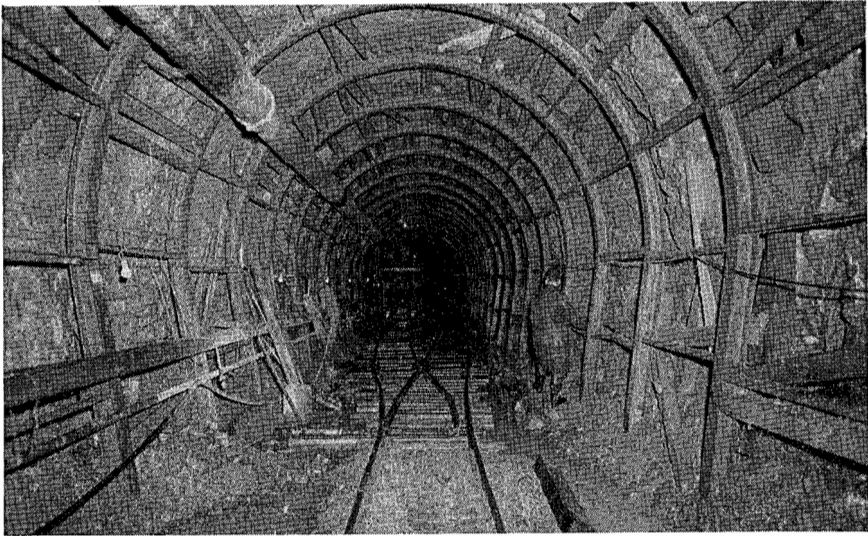
FIG. 11.—LOOKING SOUTHERLY FROM STATION 7 + 65 NEAR SOUTH END OF LONG SECTION OF STRUCTURAL STEEL. ROCK IS ARGILLITE OF CAMBRIDGE FORMATION IN IMMEDIATE FOREGROUND; ROCK IS DIABASE FURTHER SOUTH
