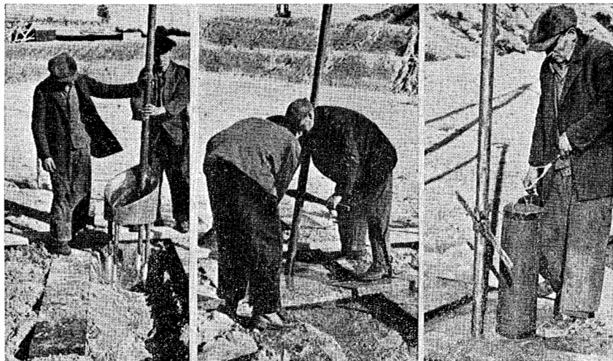
FIG. 14.—ECCENTRIC JETTING DEVICE IN OPERATION
