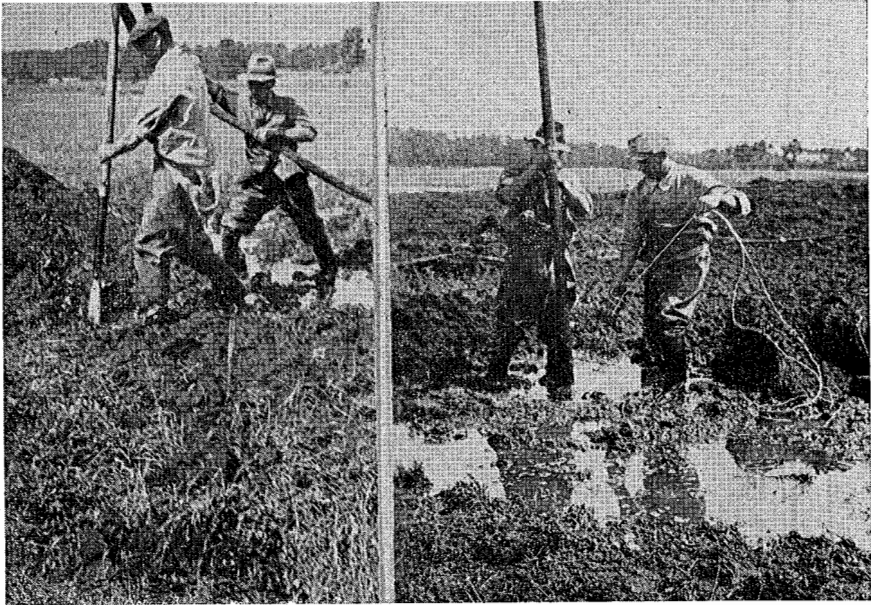
FIG. 5.—JETTING OF SMALL CHARGES TO BREAK UP SURFACE MAT OR CRUST
