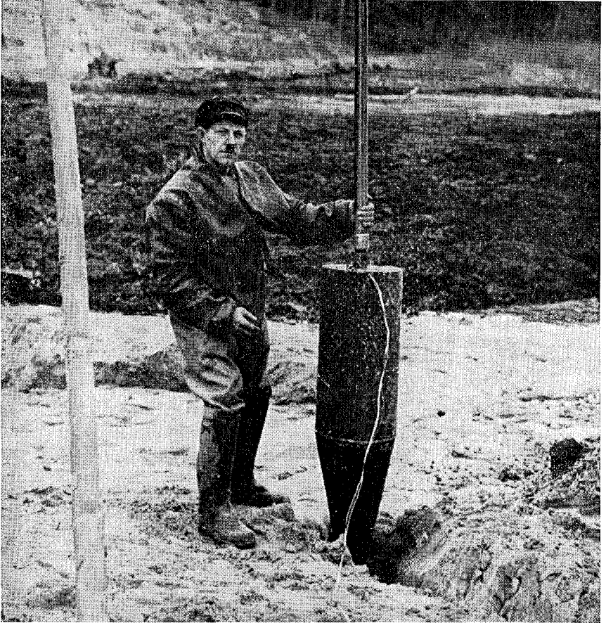
FIG. 13.—TORPEDO CHARGE READY TO BE JETTED THROUGH FILL
