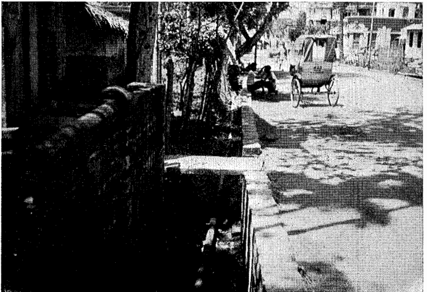
FIG. 6.—WATER MAIN LAID IN DRAINAGE DITCH
