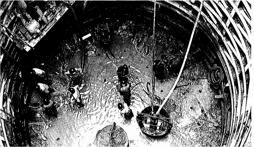
Fig. 22. — Sinking Shaft 7B. Has reached elevation +48 feet. 8/24/48.
