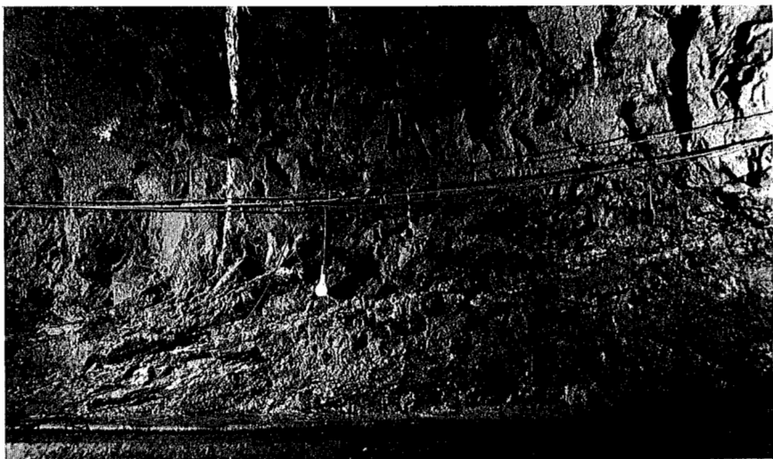
Fig. 17. — Station 112 + 25, north wall. Contact of conglomerate with overlying melaphyre. Apparent dip 25^{\circ}W .
