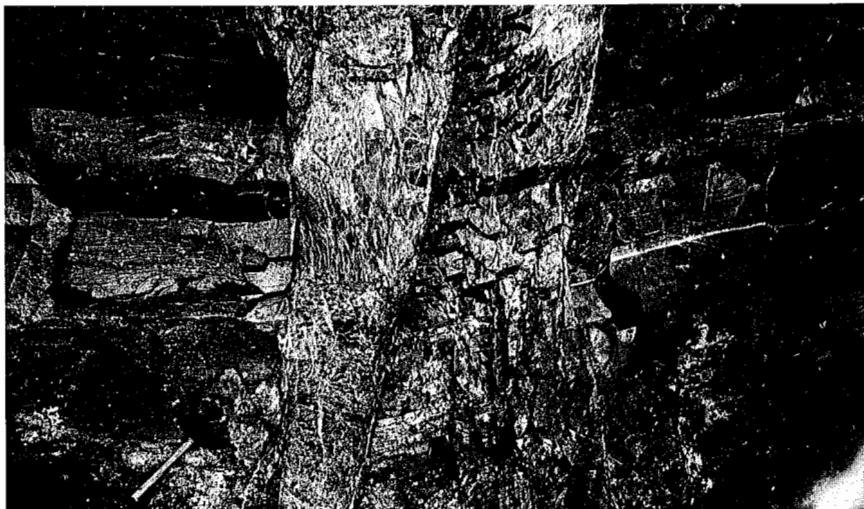
Fig. 18. — Station 285 + 06, north wall. Fault zone several feet wide; left part is a breccia, right part is fractured argillite. Country rock is argillite. On left side of fault the bedding strikes parallel to the tunnel and dips gently north. On right side of fault the strike of the bedding is diagonal to the tunnel and dips gently northwest. The fault-trace separation along the fault appears to be very small. 1/21/49.
