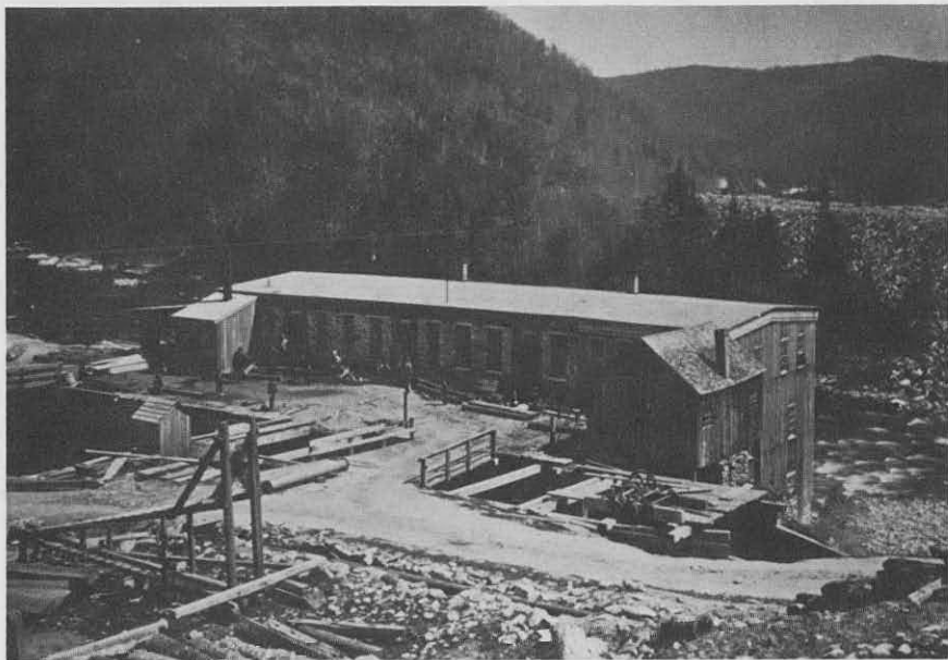
Machine shop near east end of tunnel. Note "muck" pile in the background.
