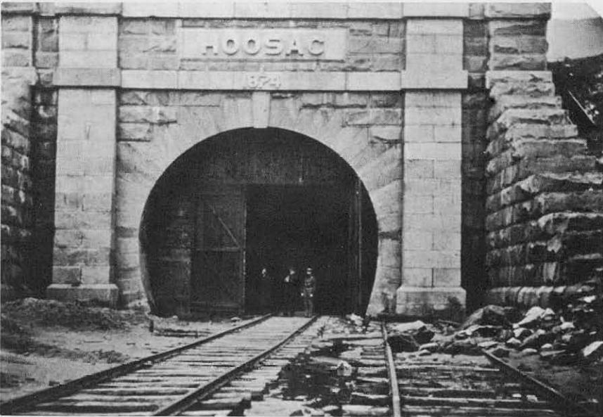
Famous West Portal of the Hoosac Tunnel constructed by Francis and Walter Shanly in 1874.
