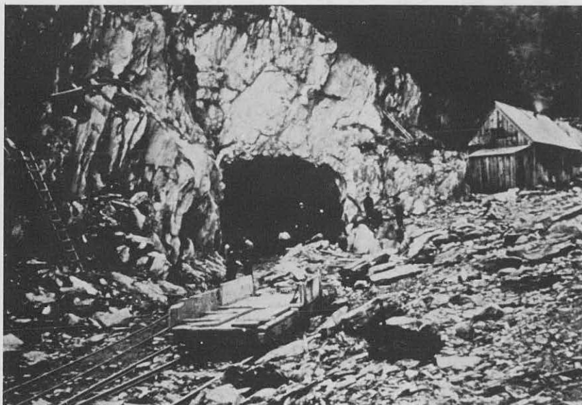
East end of Hoosac Tunnel during construction. Portal erected here in 1877 by B. N. Farren.
