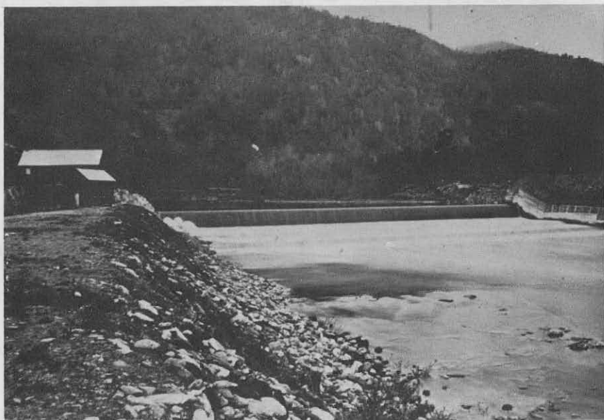
Famous Deerfield Dam constructed under supervision of Thomas Doane, Circa 1864.
