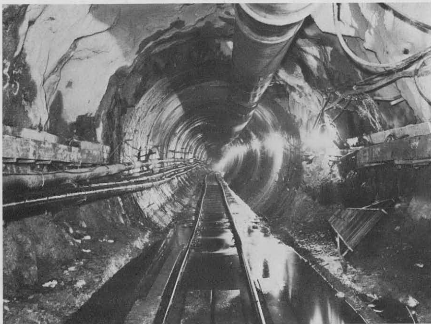
Figure 7: View southeasterly from shaft 7C into the Mole-driven section of the tunnel. The rock is Cambridge argillite.
