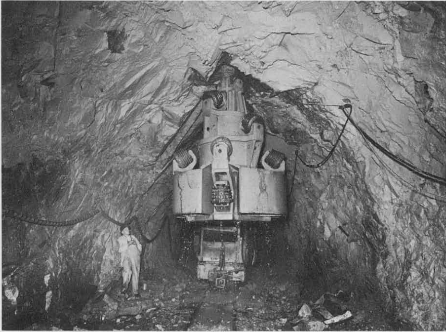
Figure 9: Raise drill being lifted into position at shaft 7D.
