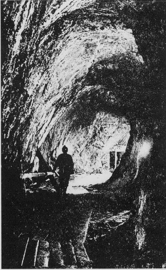
Figure 5: Tunnel Excavated by Fire Setting
