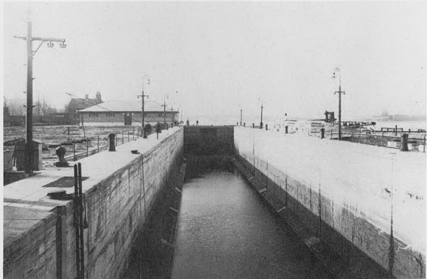
Sluices under construction, upstream face, June 1907. (From MDC files).
