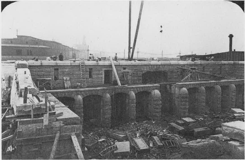
Completed lock, 1909. (From MDC files).
