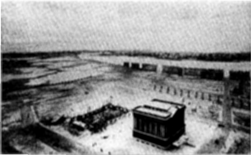
Figure 2. Diorama looking northwest across the Back Bay filling towards Cambridge. The Rogers Building is shown under construction in the foreground.
