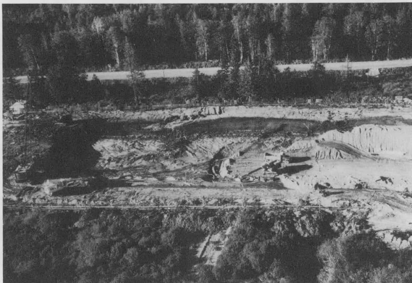
FIG. 16. POST-TREATMENT EXCAVATION AND BACKFILLING OF CUT FOR CANADIAN PACIFIC RAILWAY
