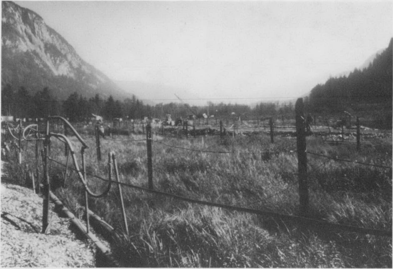
FIG. 15. ELECTRODES INSTALLED FOR CANADIAN PACIFIC RAILWAY CUT
