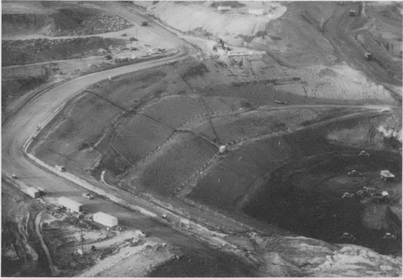
FIG. 17. 200-FT HIGH EXCAVATION SLOPE IN STABILIZED SILT, REVELSTOKE DAM
