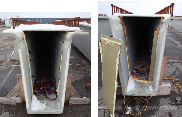
Figure 22. Instrumented FRP composite bridge girders
