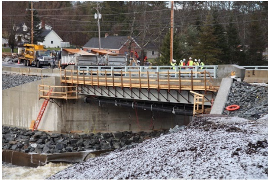
Figure 26. Constructed Grist Mill Bridge.
