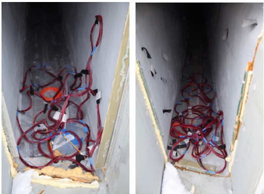
Figure 25. Instrumented FRP composite girders 3 and 5.
