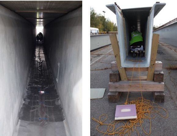
(a) Installed textile. (b) Epoxy container. Figure 20. Installation procedure – Step 5).
