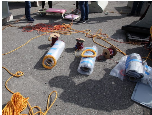
Figure 16. Installation cart and three sensing textile rolls.
